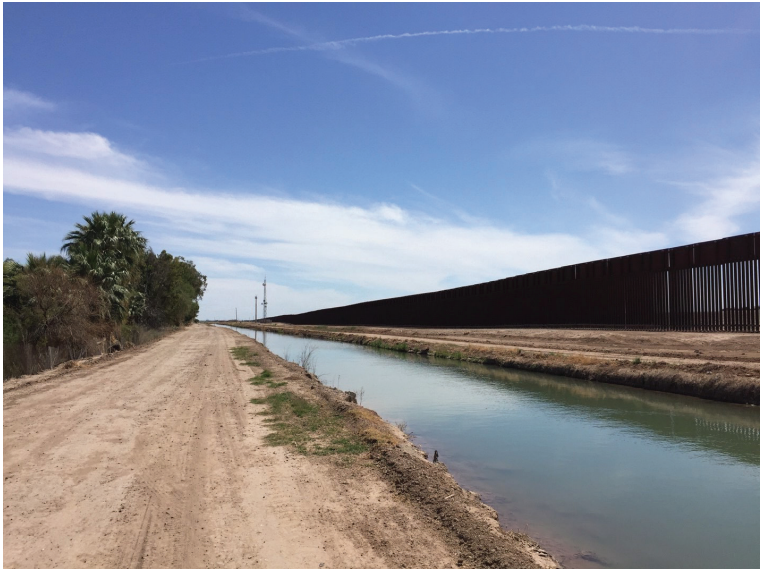
Border wall between Gadsden, Arizona, and Baja California State, 2016
