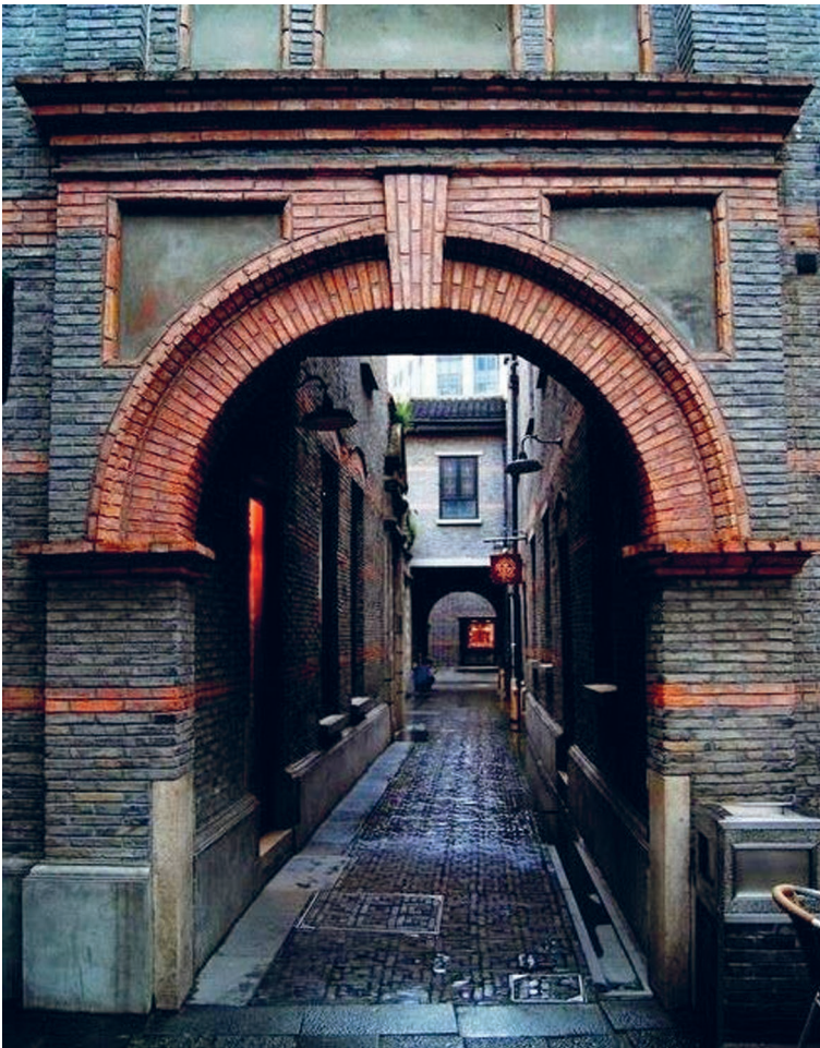
Photo 6. Red brick used for an arch and in accents, Xintiandi (Tina Kanagaratnam)
