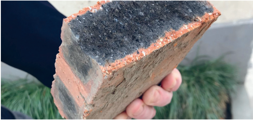
Photo 3. Under-burnt brick, Shanghai 2018 (Tina Kanagaratnam)
