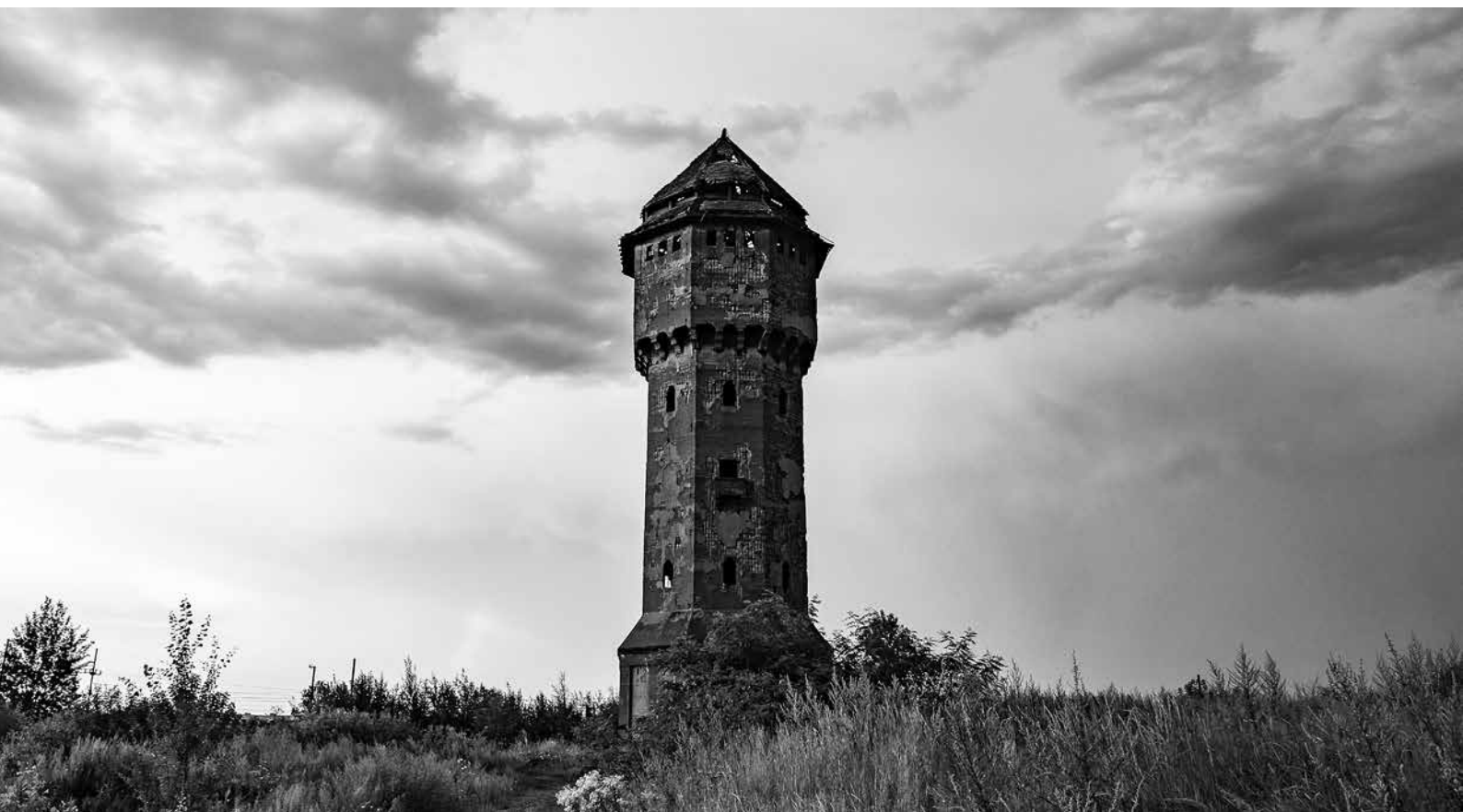
Water tower belonging to the former Uthemann Zinc Smelter in Katowice-Szopienice | Photo: Rafal Opalski
